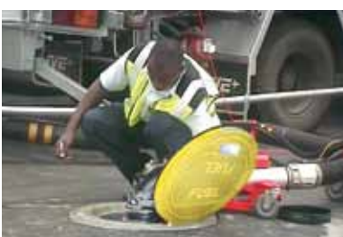
Waterproof cover and frame assemblies with either aluminium or composite doors prevent fluids and debris from entering the pit when the cover is closed.
